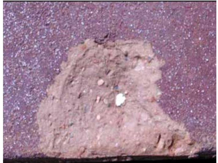
**Strength and durability** of brick are not affected by lime pops, but they can be aesthetic issue, if they occur in sufficient size and number as to detract from the appearance of the wall. All Acme brick are manufactured to meet the requirements of *Standard Specifications for Facing Brick*, ASTM C 216, Grade SW, for exposure to "severe weathering." **We warrant the brick to perform accordingly for 100 years.**
