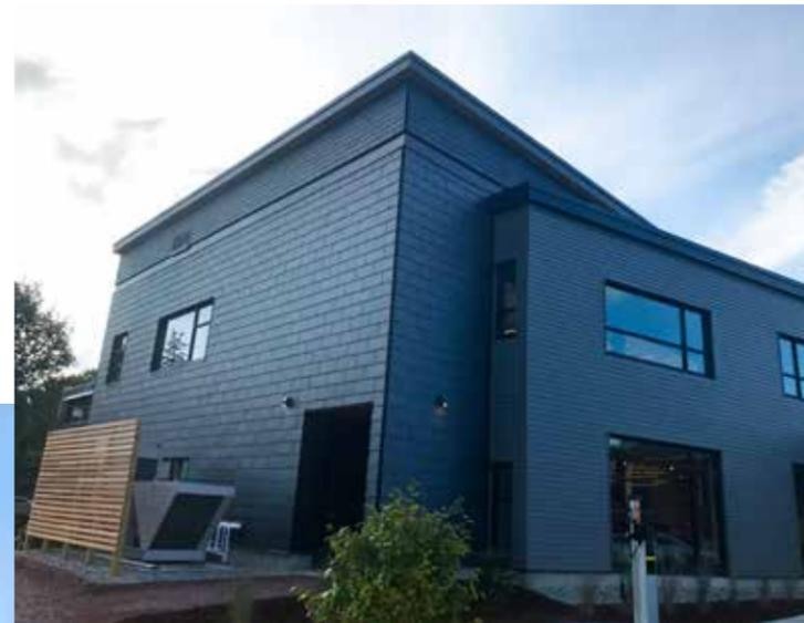
“One major challenge was because the walls of the library were tall, we were apprehensive about load bearing factors. And because the building was designed with a Net Zero energy, exterior envelope of 4” thick insulation, the weight of the façade was a concern,” Nedzinski continued. “The installation process was researched, and ultimately by crossing layers of z-girts, the CupaClad® system was successfully adhered to the building’s exterior.”
