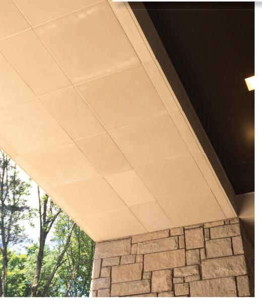
Completed in 2014 this LEED certified building sports a 645 sq ft RockCast cast stone soffit of 194, 1.5" thick panels. Twenty different panel sizes were needed, ranging from 1' 11.625" x 1' 11.655" to 7.625" x 1' 11.625", as well as 6 unique trapezoid shaped panels. The new headquarters, referred to as the "Store Support Center," brings almost 900 employees for the country's largest operator of retail farm and ranch stores under one roof.
