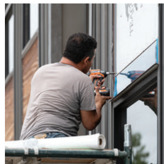
initial panel install
