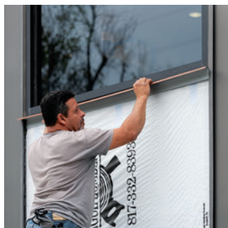
header install over vapor barrier
