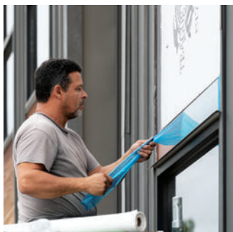
removal of protective film
