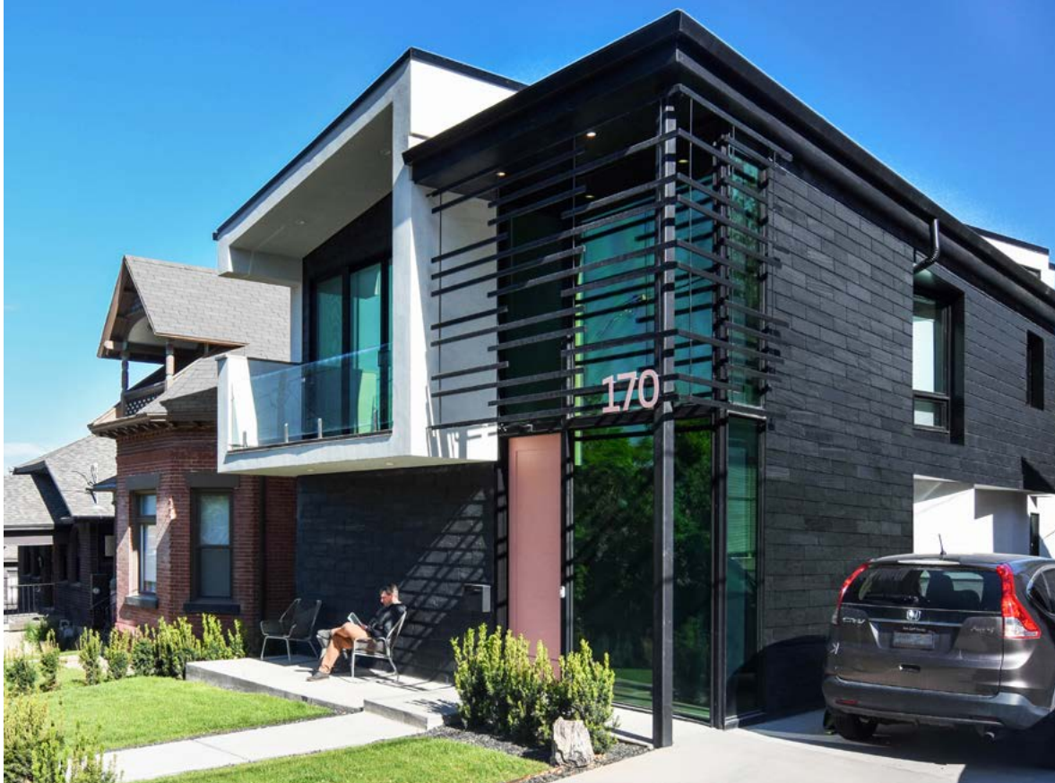
Shama House, Utah / CUPACLAD Logic
