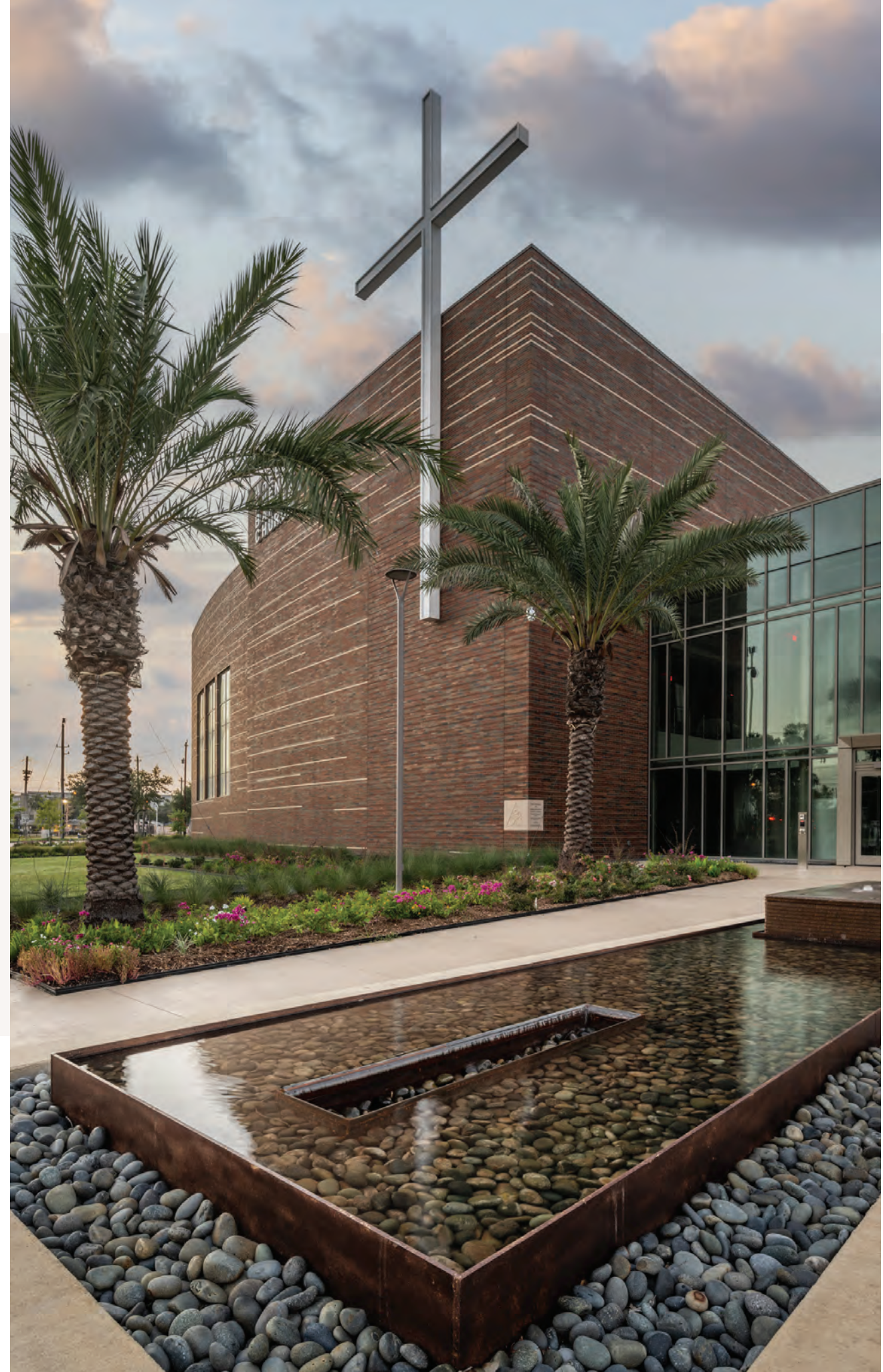
Wheeler Avenue Baptist Church in Houston uses a mix of colors, including white and black brick, in its design by Perkins&Will.
